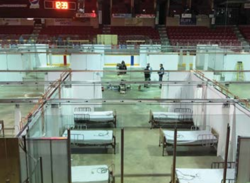
View of the field hospital under construction.
