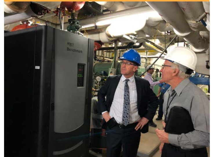
Local MPP Bill Walker tours boiler room with GBHS Engineering staff.
